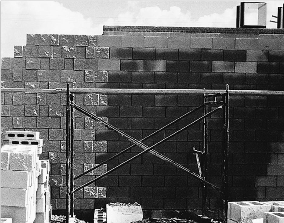
Figure 2: Normally, splitface CMUs are more prone to wicking than standard CMUs. With DRY-BLOCK® throughout, the splitface CMU repels moisture and dries out rapidly after a rain; the standard CMU remains moisture saturated.
